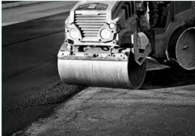
Figure 16.2. Roads are often paved with refined bitumen, which is derived from crude oil. Thus, the cost of paving roads varies with the price of oil, and the short-term volatility of oil prices presents challenges for pricing contracts for long-term construction projects such as paving roads.
